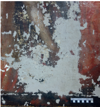
Fig. 218: Same detail after filling
