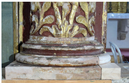
Fig. 173: During formal reconstruction with massive wood
