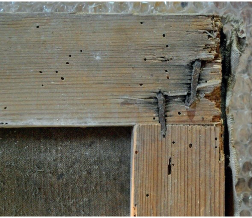
Fig. 193: Reworked corner joint
