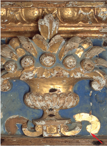
Fig. 25: Even before gilding, the lower right volute had broken off. Here, the gilding lies on the flat support (condition before treatment). The blue paint has a patchy, irregular appearance
