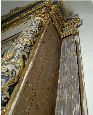
Fig. 89: Bare wood on the side of the retable; condition as found
