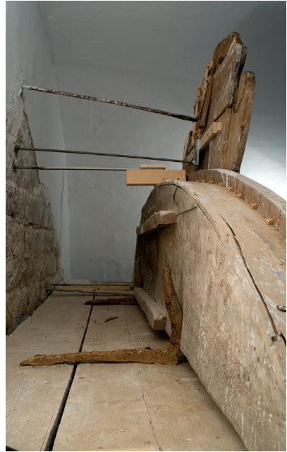
Fig. 102: Condition after treatment; the original mounting with two naturally grown wooden "knees" and one iron strut is reinforced with two additional stainless-steel struts; small wooden blocks stabilise the outer moulding
