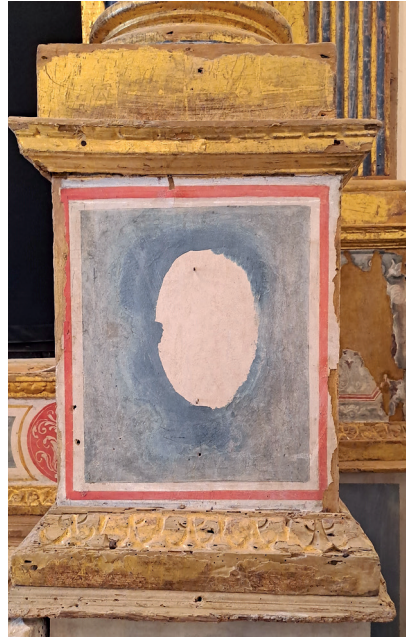
Fig. 74: Right postament; empty position of former attached cartouche
