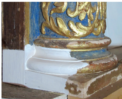
Fig.176: Reconstructed area with preparation
