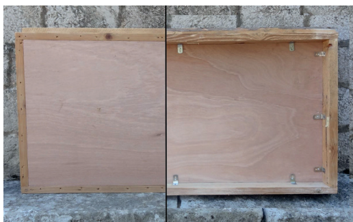
Fig. 215: Strainer box with backboard protection; front (left) and back (right)
