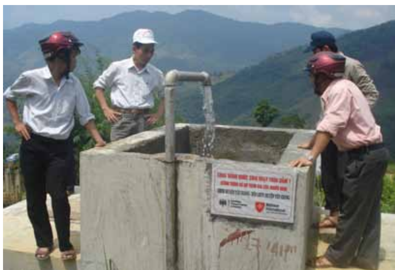
Handing over of water supply system to community in Abanh 2 village, Trhy commune, Tay Giang District, Quang Nam Province, Vietnam
