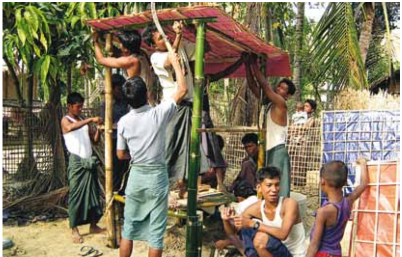
Latrine construction, Myanmar
