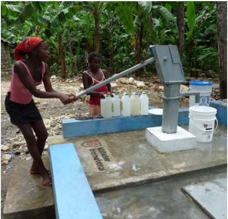
Well constructed in Darbonne, Haiti
