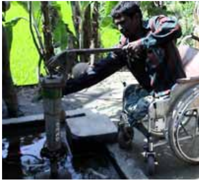
Person with disability using pump installed at the edge of the apron 96
