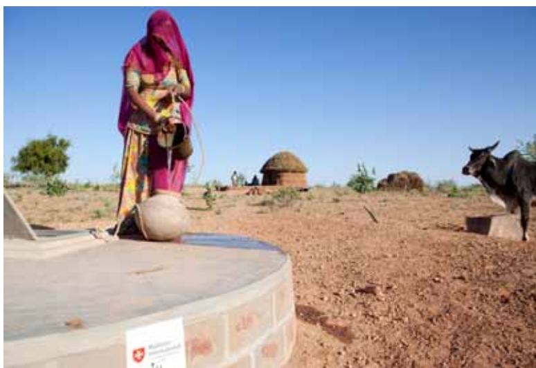
Rainwater harvesting in underground tanks, Rajasthan, India CARMEN WOLF
