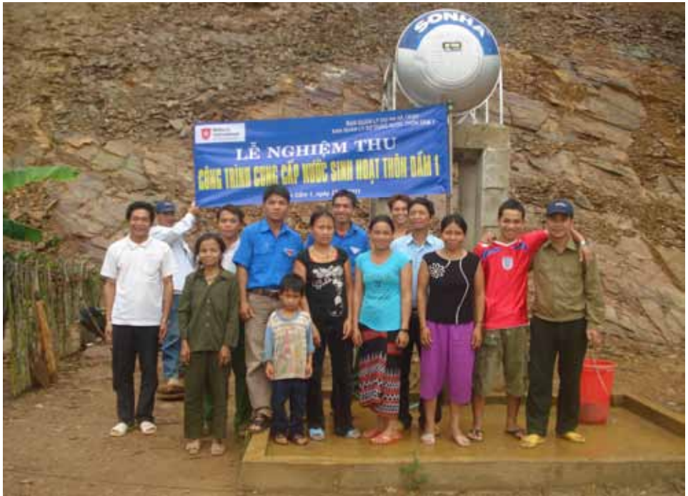
Villagers trained to do repairs and maintenance for water supply system, Vietnam
