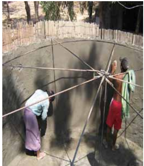
Ferrocement tank under construction for school in Myanmar
