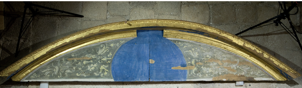
Fig. 80: Pediment with blue circle hidden behind the cartouche (here removed), condition as found
