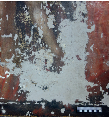
Fig. 218: Same detail after filling
