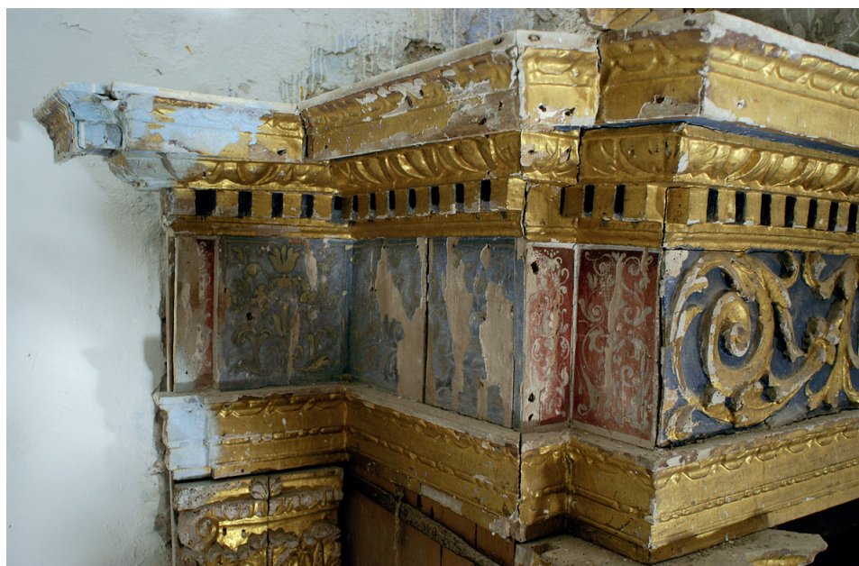
Fig. 91: Holy Cross retable; left part of the entablatura, condition as found; white paint splashes from the wallwashing on the gilding
