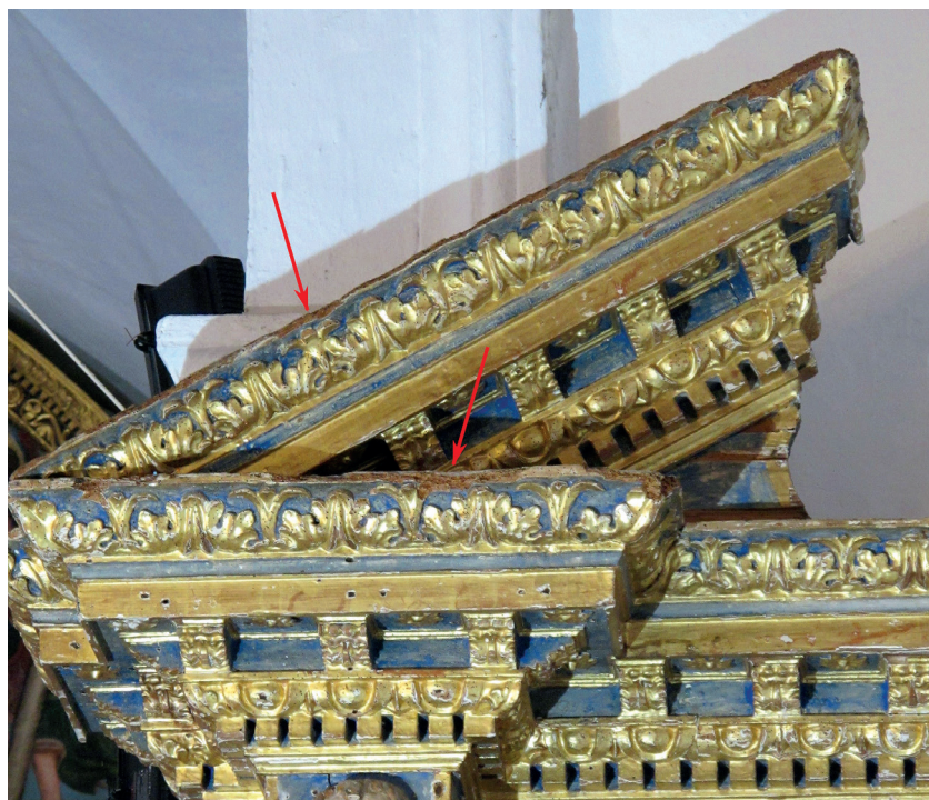
Fig. 166: St Mary retable; condition as found; losses in the outer contour
