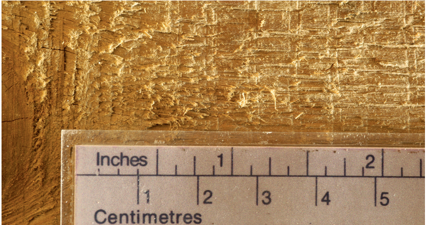
Fig. 21: Marks of mechanical sawing
