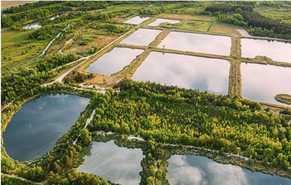
Figure 15 Wet Retention Ponds in Agricultural Lands Source: (BTL LINERS, n.d.)
