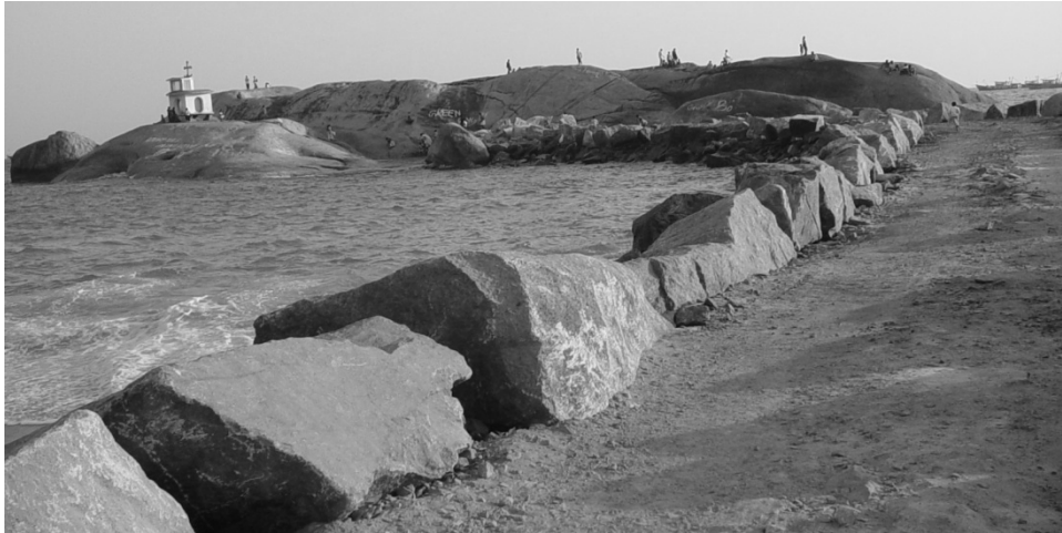
Figure 5: Groyne at Simon Colony (designed so that the natural outcrop acts as a head) Source: Sundar & Sundaravedivelu (2007)
