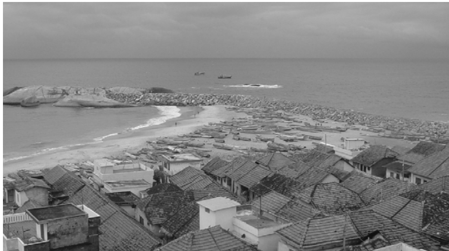
Figure 8.a: Groin serving as a coastal protection measure as well as boat landing facility Source: Sundar & Sundaravedivelu (2007)
