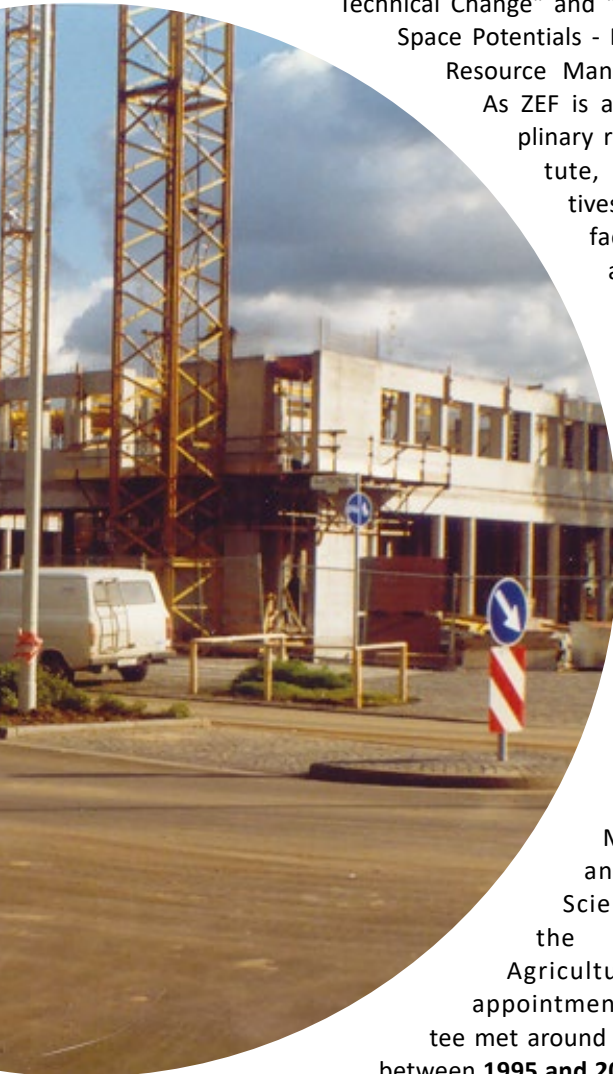
ZEF: A building construction site 1989
