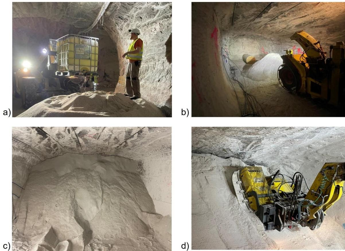
**Fig. 2.13** Construction process of the KOMPASS backfill body. a) Wetting of the KOMPASS material. b) Emplacement of the dry crushed salt backfill. c) KOMPASS backfill body before densification. d) Densification process of the KOMPASS backfill body /SCH 23/
