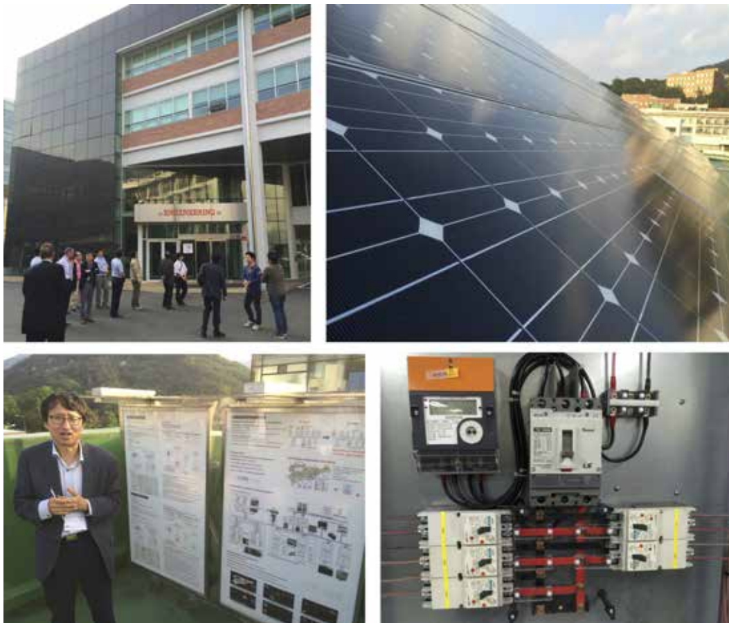
Figure 8.7 The 1970 Engineering Building at Seoul National University (top left), was completely remodeled in 2012 to become energy-efficient. It is equipped with a 36 kW-peak PV system (top right). Prof. S. Sul explains the 380 Vdc power line to which EV chargers, all electronic loads and the AC distribution system are coupled (bottom left). The 380 Vdc system is electronically protected and also has 380 DC circuit breakers (bottom right) (pictures taken by Prof. De Doncker, with permission of Prof. Sul).
