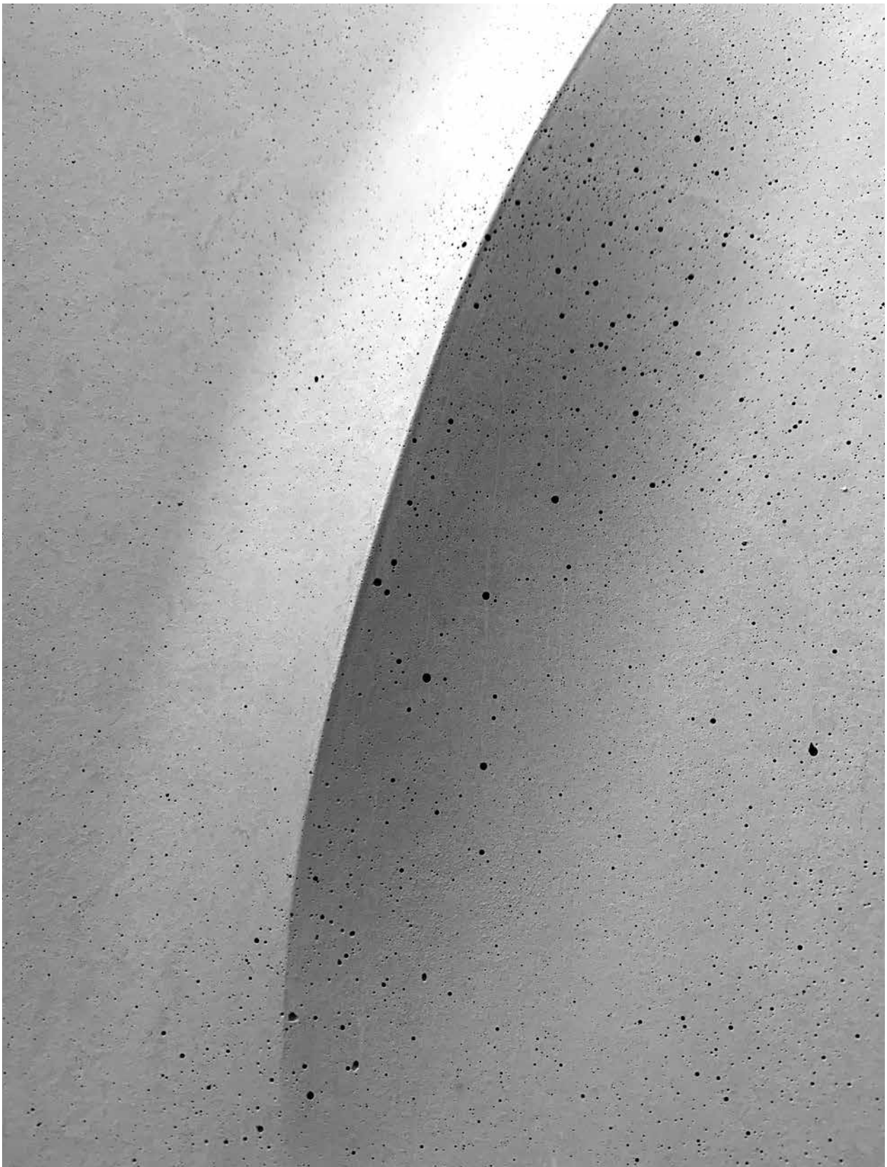
Abb. 159: Detail Betondemonstrator (Runkel)
