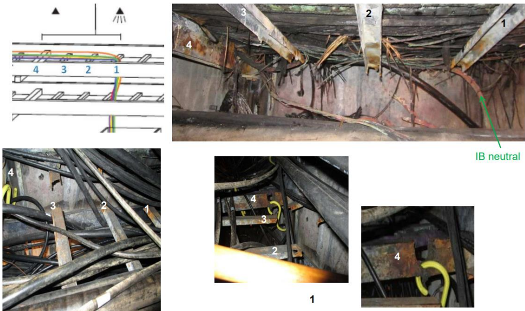
Figure 3 Cable trays damage evidence [3]
