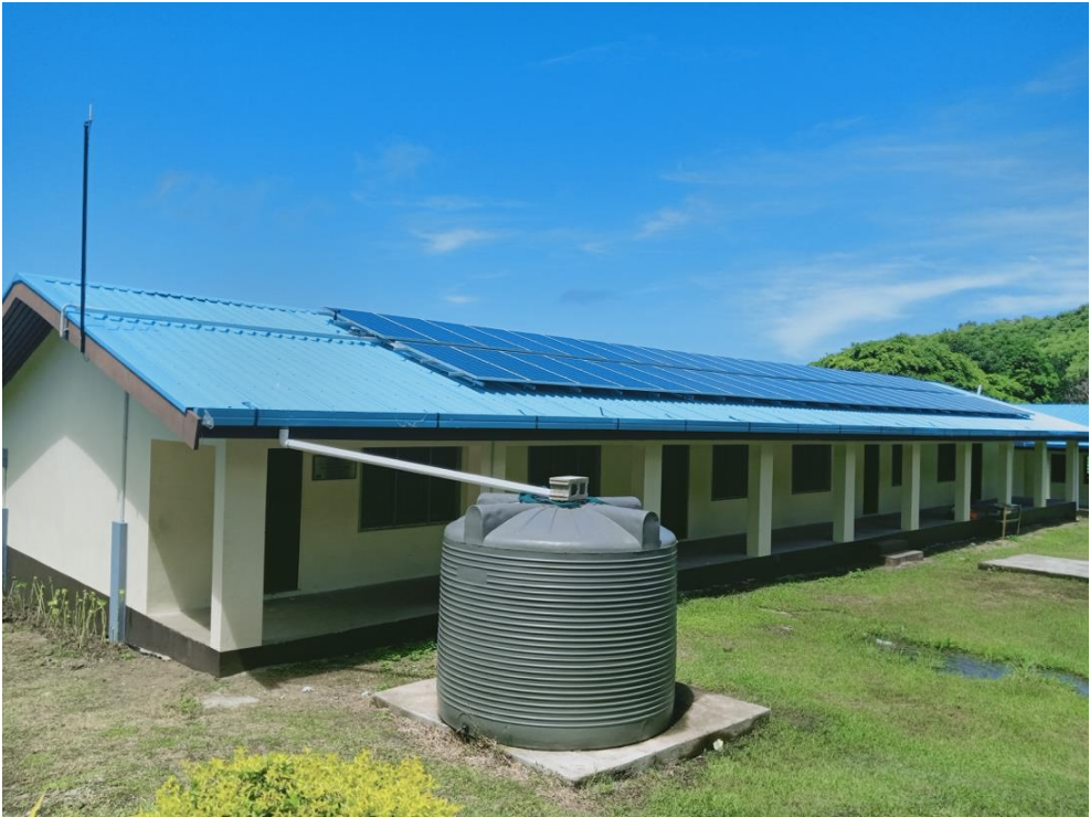
Photo 5: Water-storage tank and solar PV panels at Yasawa High School (Fiji)
