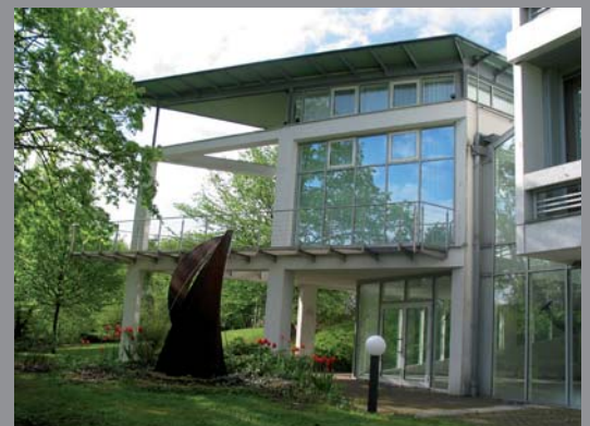
B-IT main building.
