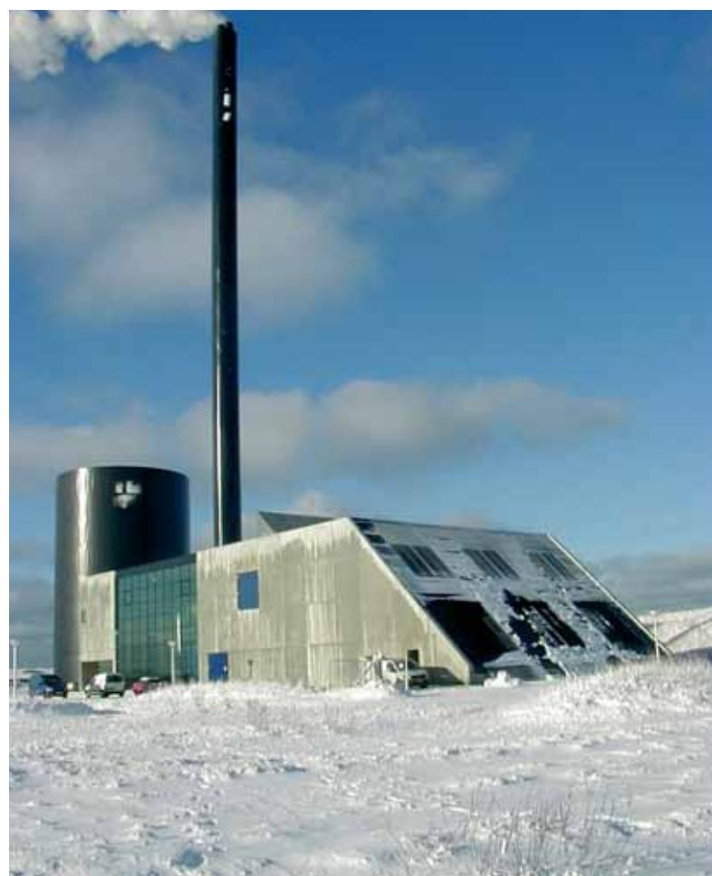
Figure 3: CHP plant with heat storage in Skagen
