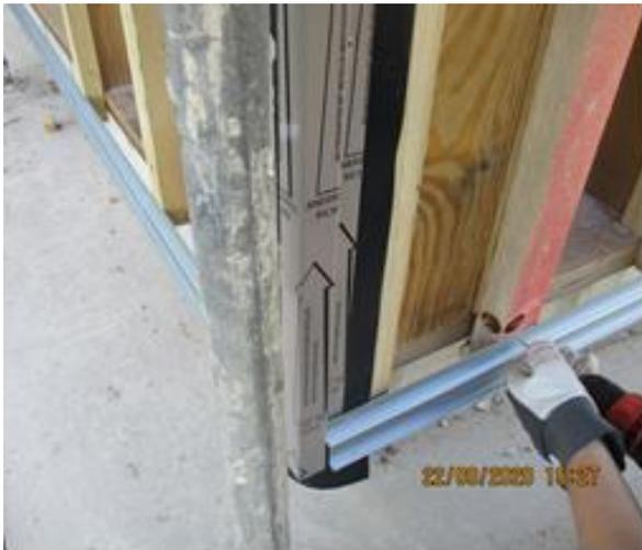
Bild 234 *Demontage der Systemprofile*
