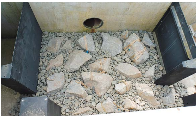
Sohlsubstrat in der FAA Malliß
