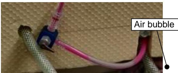
**Fig. 4.50** Air in the injection tubing
