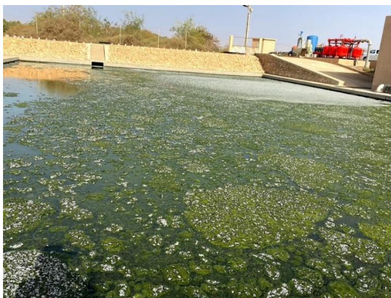
Photo 5: The finished treatment plant in Tiznit, organisational issues have prevented the use of the plant as algae grow in the sandfilter (Source: El Meknassi, 2020)
