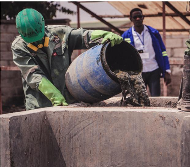
Above: Sludge from a pit latrine with relatively low moisture content being disposed of at a treatment facility in Lusaka
