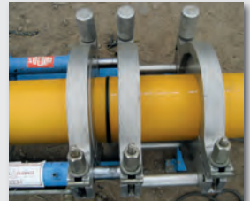
Figure 9: heating element butt fusion
