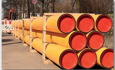
Figure 5: Pipes in rods
