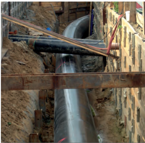
Figure 13: installation in a trench with sand bedding
