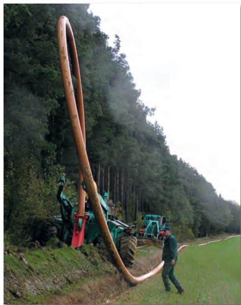
Figure 18: plowing method
