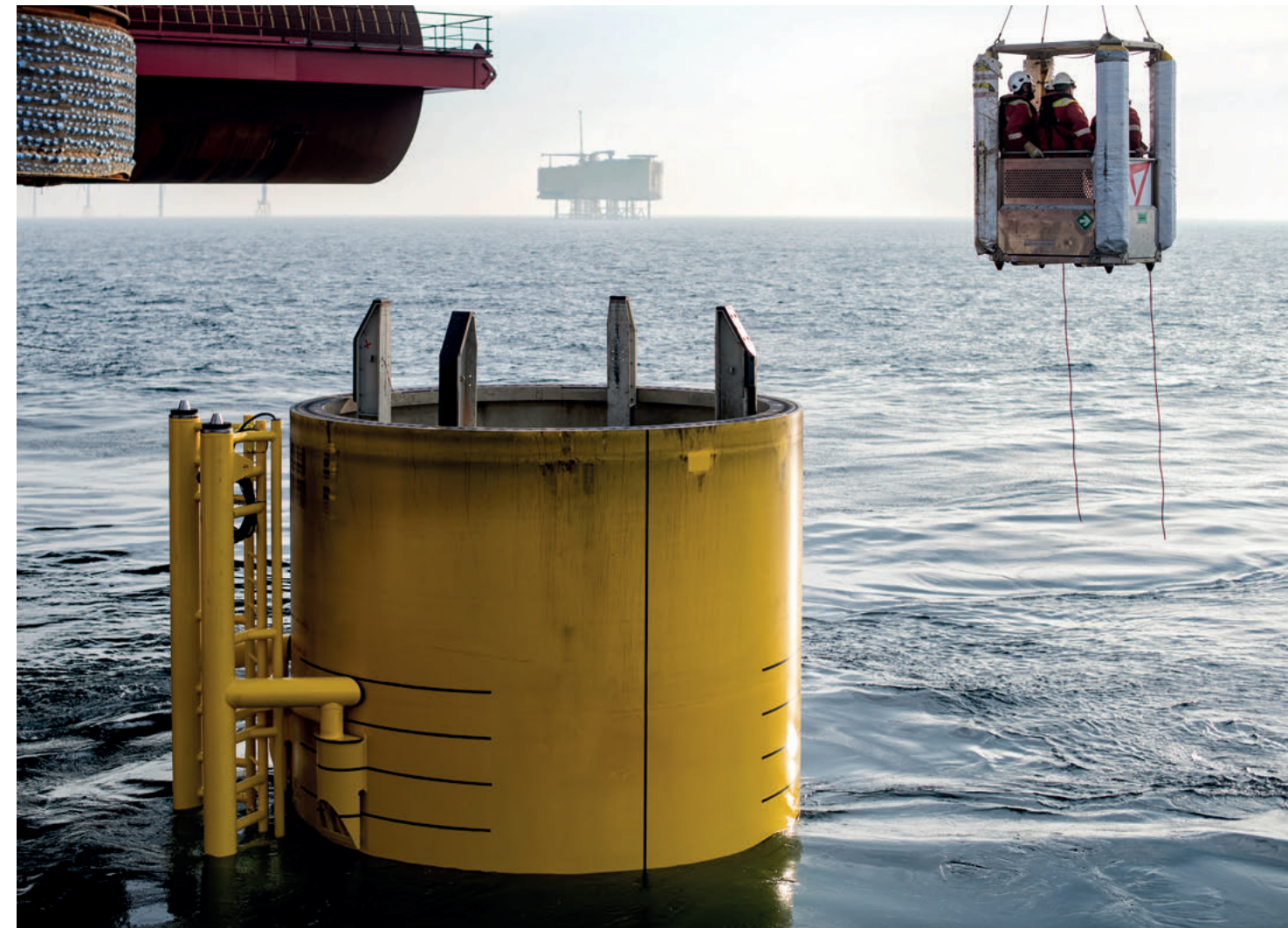
Trianel Windpark Borkum II: Monopile
