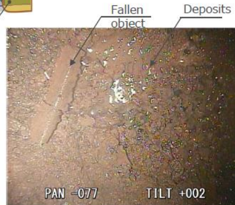
Photo location B Bottom of pedestal
