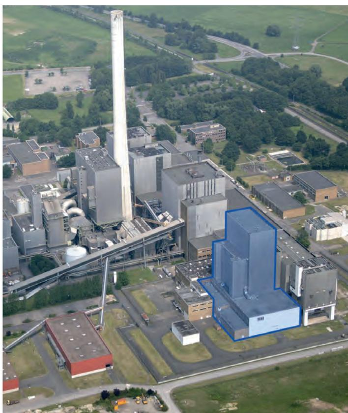
**Fig. 11:** Building of the THTR-300 (area of safe enclosure blue-coloured)
