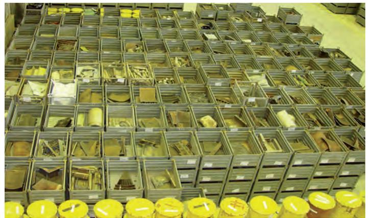
Fig. 33: Boxes with sorted residues for clearance
