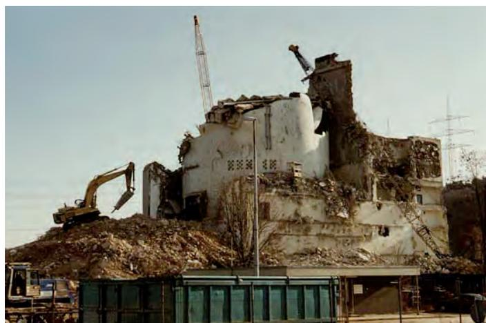
**Fig. 17:** Conventional demolition of the outer building shell of the Niederaichbach nuclear power plant
