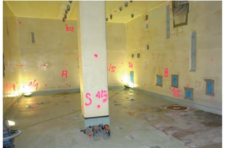
Fig. 36: Room with markings to determine surface contamination
