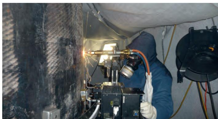
*Fig. 28: Manual use of thermal disassembly techniques*
