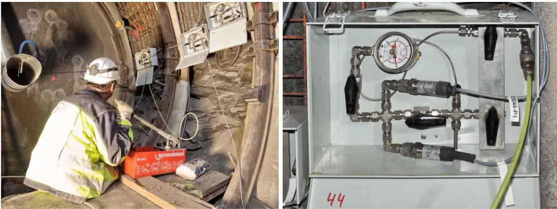
**Fig. 5.17** Installation of the transducer racks in the rear part of the tunnel
