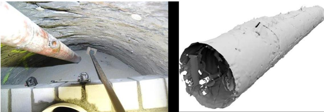
**Fig. 5.7** Left: Granular buffer emplacement using an auger system, right: 3D image of the microtunnel test section before installation for volume calculation /GAU 14/
