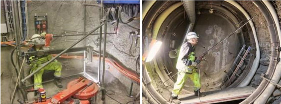
**Fig. 5.16** Drilling of the minipiezometer boreholes: tunnel front (left), radial borehole at the tunnel rear (right)
