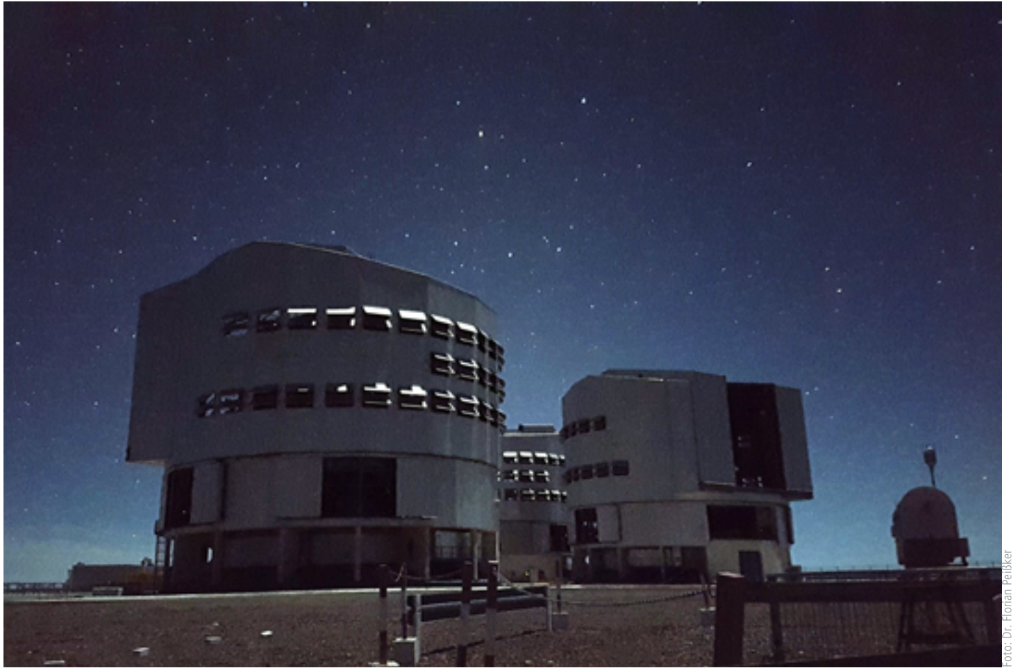
Very large Teleskop in Chile
