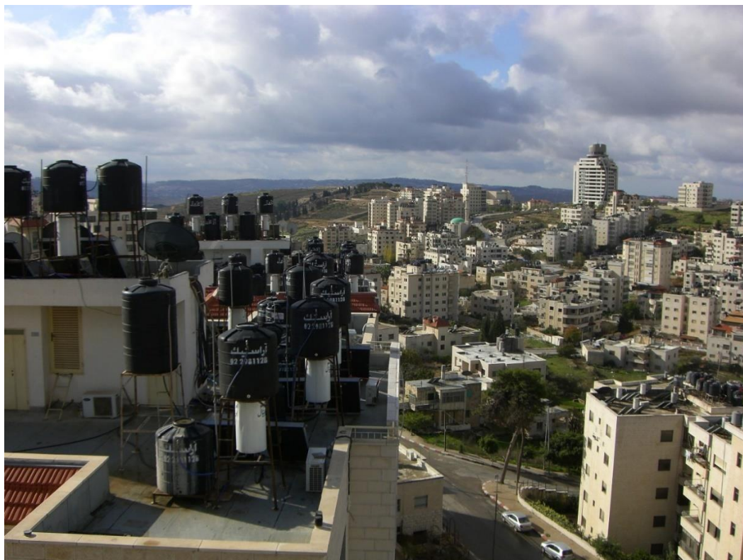
Water reservoirs on roof tops in Ramallah serve to bridge gaps in water supply and balance variations in water pressure
