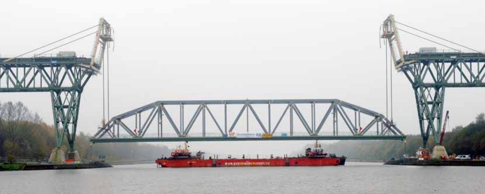
Inserting the middle section of the high-level railway bridge at Hochdonn.
