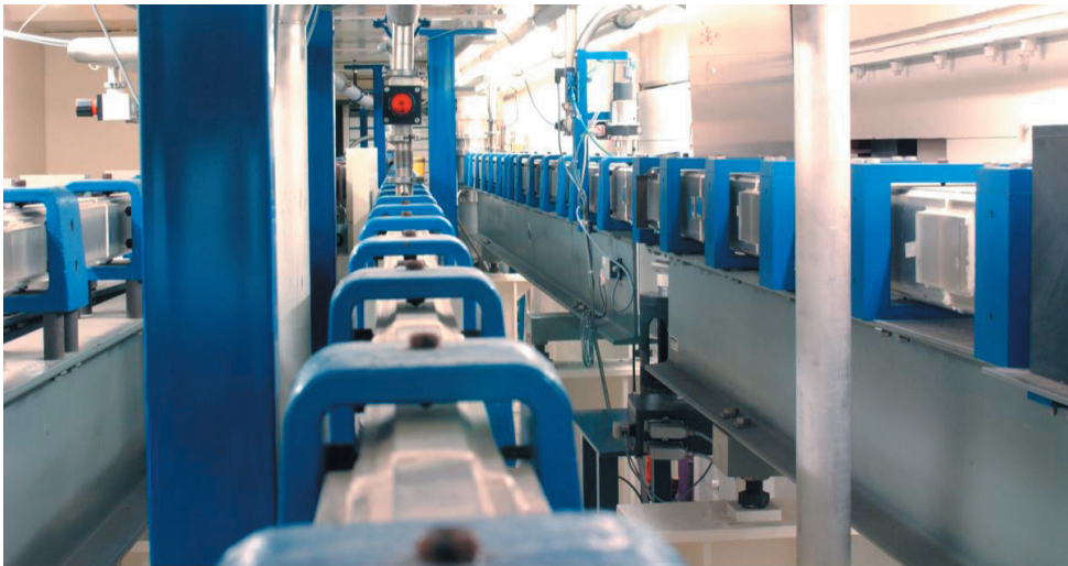
Fig. 7: Neutron guides serving the cold neutron instruments at the former FRJ-2 research reactor in Jülich.
