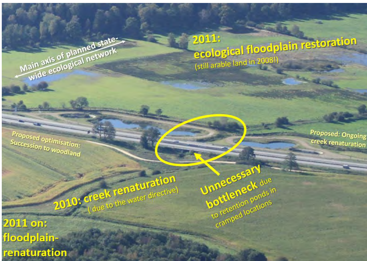
Fig. 40: Artificial bottleneck at a water course passage and compensatory habitat enhancement
