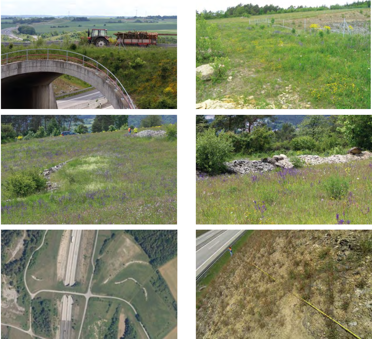
Fig. 44: Complementary solutions (joint-use structures, integration of mitigation and offsetting measures, and appropriate landscaping of verges)
