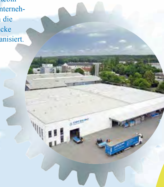
Röchling Logistik-Center in Troisdorf
