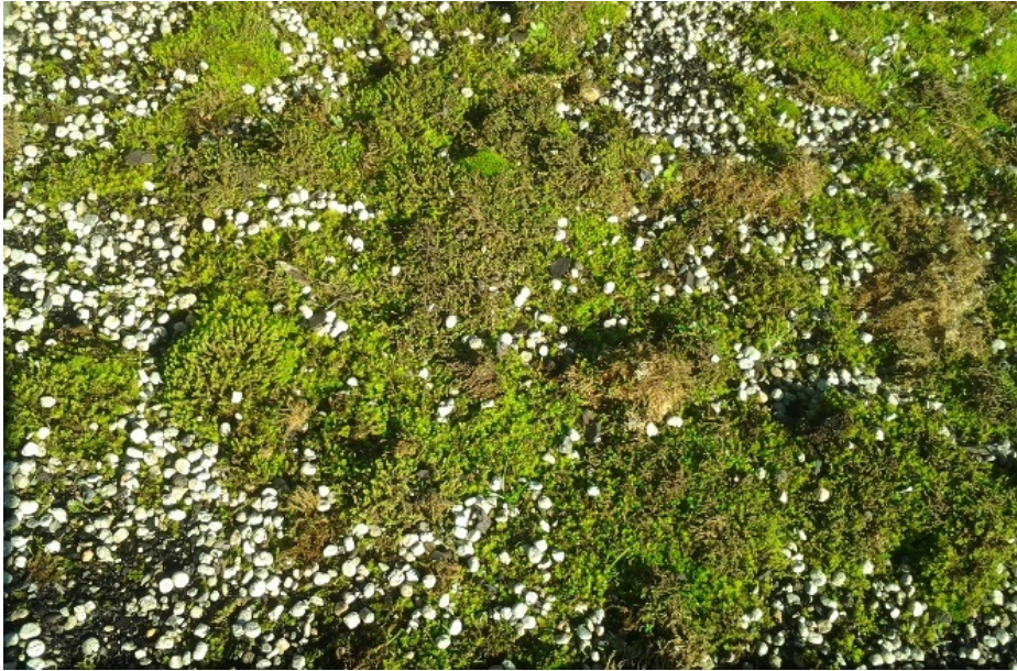
Figure 1: Green roof based on moss-dominated biological soil crusts (Biocrusts) (Image: Ricardo da Cruz de Carvalho).
