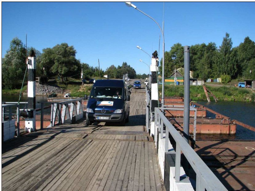
Photo 3 : New pontoon bridge crossing the Sozh river, on the road from Korma to Volincy (2013)
