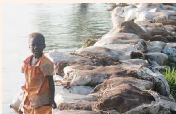
122: A sand dyke built by the village of Ere to protect against flooding by the Logone and its overflow to the Mayo-Kebbi, a neighbouring river in the Benue basin, Cameroon
