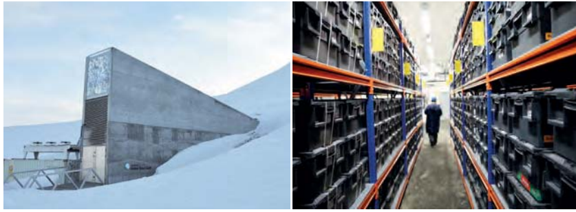
The Svalbard Global Seed Vault, half way between mainland Norway and the North Pole, is a modern-day Noah's Ark for crops. Seeds and tissue samples are stored at -18°C, in an area of permafrost without tectonic activity, 150 m inside a sandstone mountain without measurable radiation.
