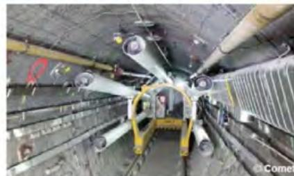
Front view of the backfilling machine in the FE emplacement tunnel
