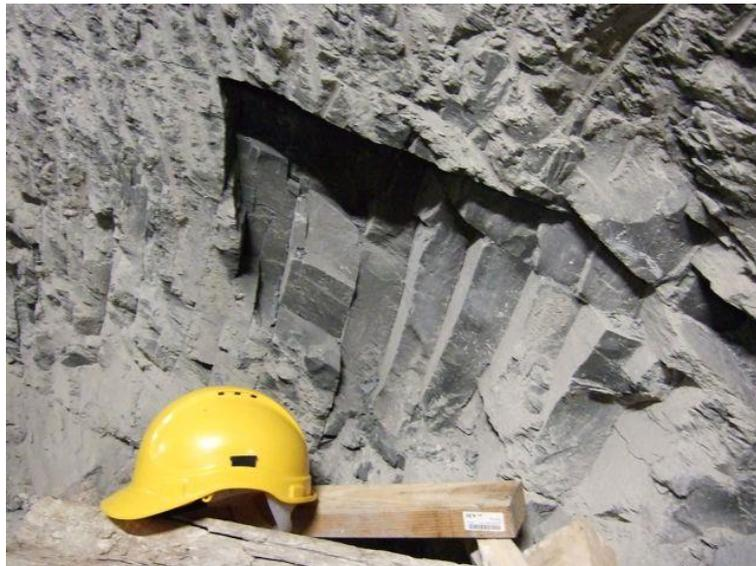
**Fig. 2.13** Example of the excavation-induced fractures, /MAD 10/ (observed during the excavation of Gallery08 as well as in the face of niche excavation; but perpendicular to the tunnel axis)
