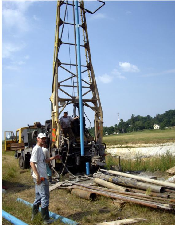
**Fig. 3.3** Installation of casing with filter sections in a borehole for its use as monitoring well
