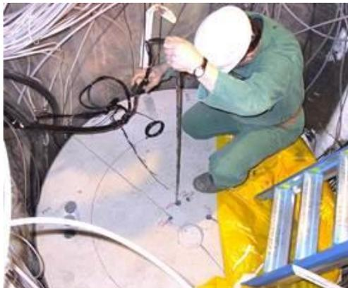
Fig. 5.11 Installation of electrode chain in the buffer at top of borehole 5
