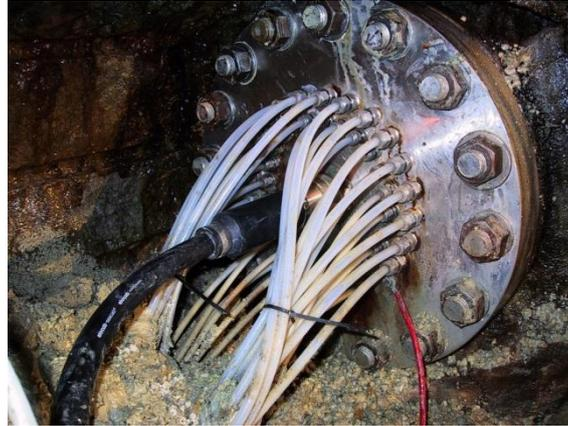
**Fig. 5.7** ELOCAB cable at head flange of a lead-through borehole
