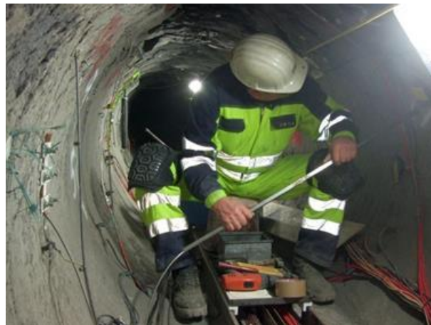
Fig. 4.7 Installation of GRS minipiezometers in the microtunnel
