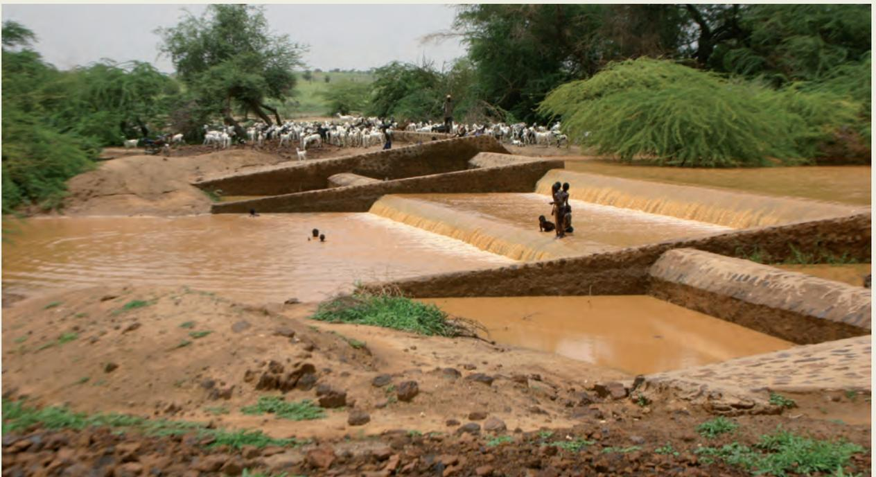
Spillway of a water-spreading weir
