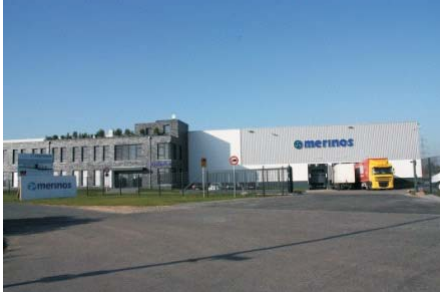
Medipa Group, Airport Gewerbepark Junkersring
