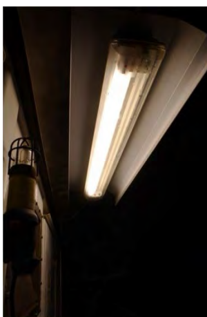
Figure 8: View of a lamp on a standby electricity generator with light guidance shield and illumination to half (Photograph: Studio B8 on behalf of RWE Dea AG).
