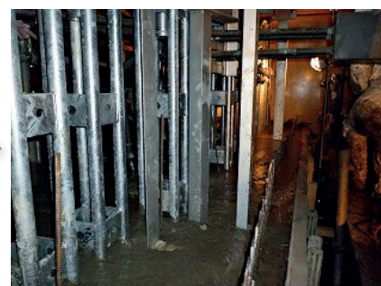
Concrete placement (pictured on July 21)
