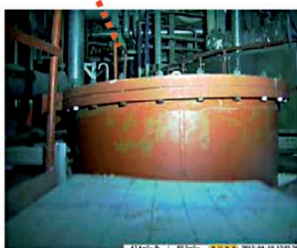
Survey inside the Unit 2's torus (April 18, 2012)
