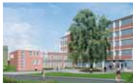
Engineering Park Aachen © AMW Projekte GmbH
